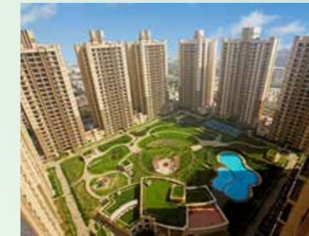
ATS ADVANTAGE PHASE I Indrapuram
